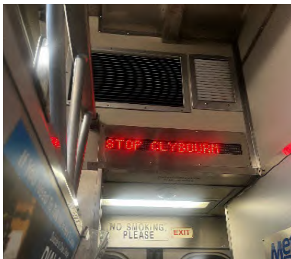
Figure 7: Interior Metra LED signage (Source: HNTB)
