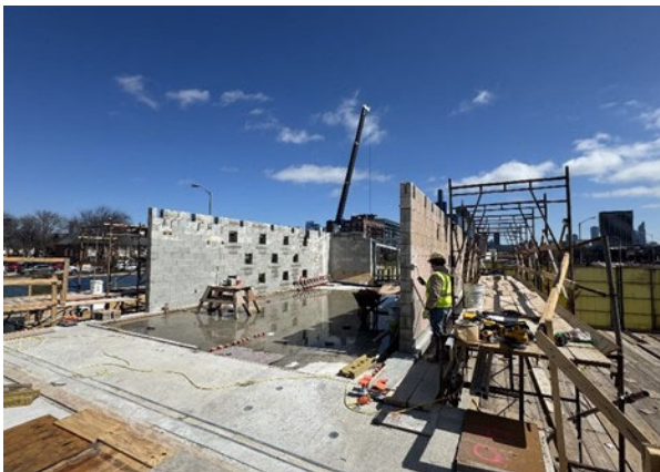
Application of vapor barrier to the Loomis Stationhouse wall.
