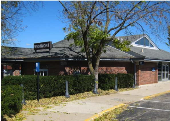
Existing Westmont Station.
