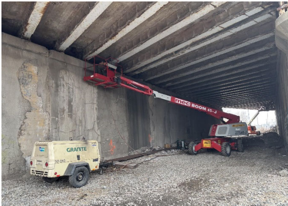
Concrete encasement removal at the EW-2 bridge.
