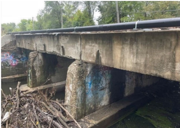
Current condition of the Stoney Creek Bridge.
