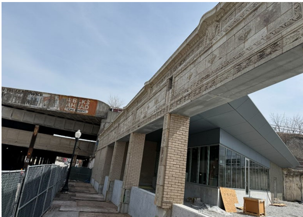
Vendor building and installed terracotta at the new Auburn Park Station.
