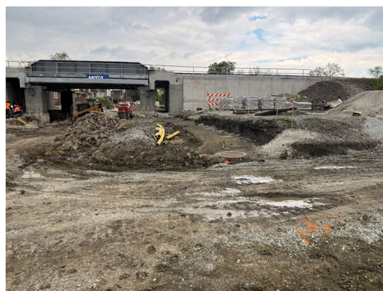
New bridge and retaining walls at Morgan Street on Metra's Rock Island District line.
