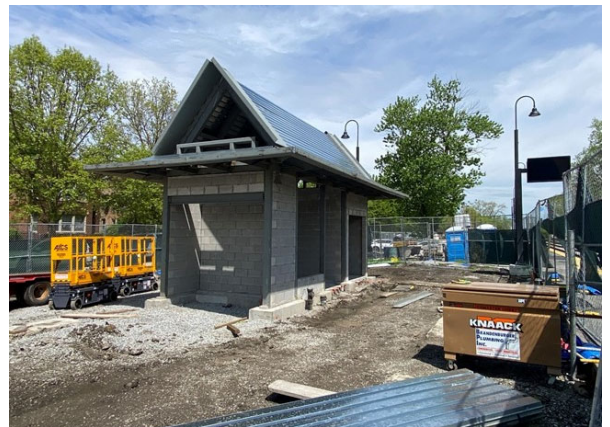
New west warming shelter at the 115 th Street Station.
