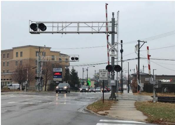
Existing Metra grade crossing.
