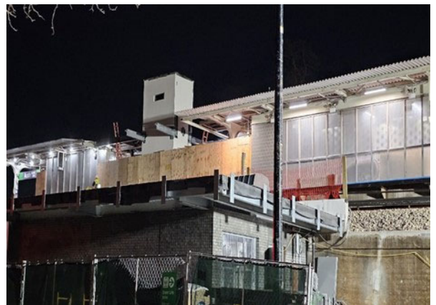
Nighttime operation – installation of steel angles on the platform at Austin Station.
