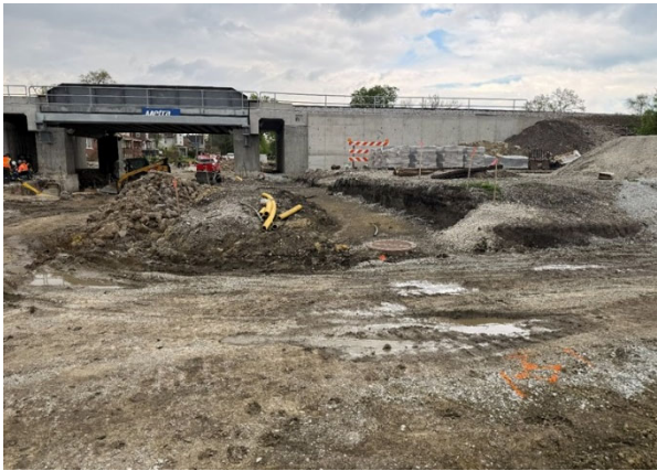
New Morgan Street Bridge.
