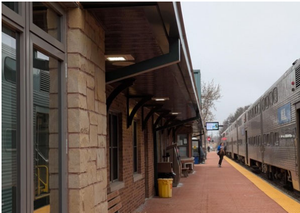
West elevation of the new building at the Fox Lake crew facility.
