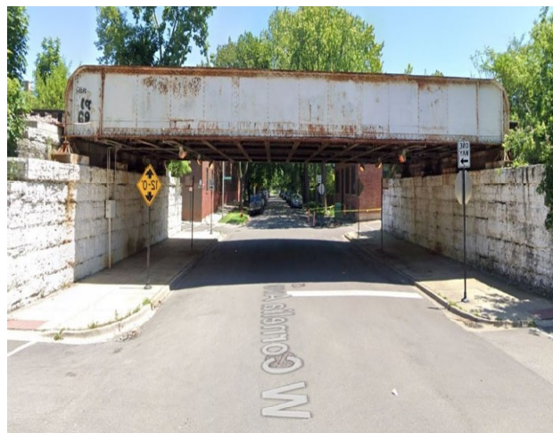
Picture of existing conditions of Cornelia Ave bridge.
