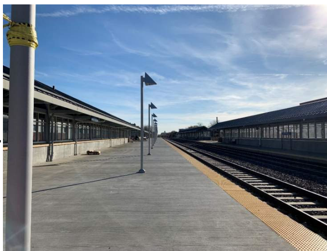
Completed platform and ADA tactile installation on track level.
