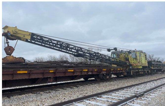
Existing Metra crane removing old ties from the right-of-way.
