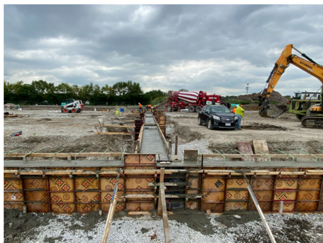
Concrete pour for the Acceptance Facility.
