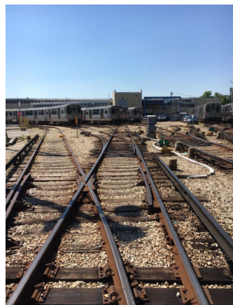
Existing Track at Des Plaines Yard.
