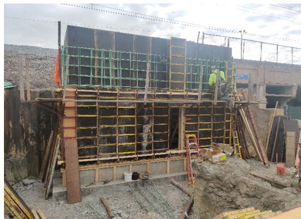
Form work for station in progress.
