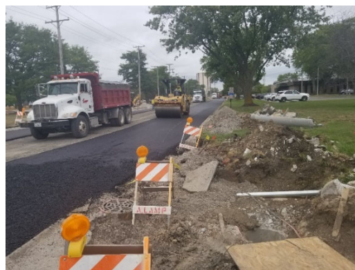
Improvements to Old Willow Road.
