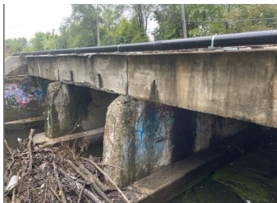
Current condition of the Stoney Creek Bridge.
