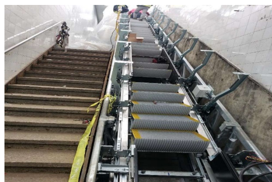
New escalator installation.
