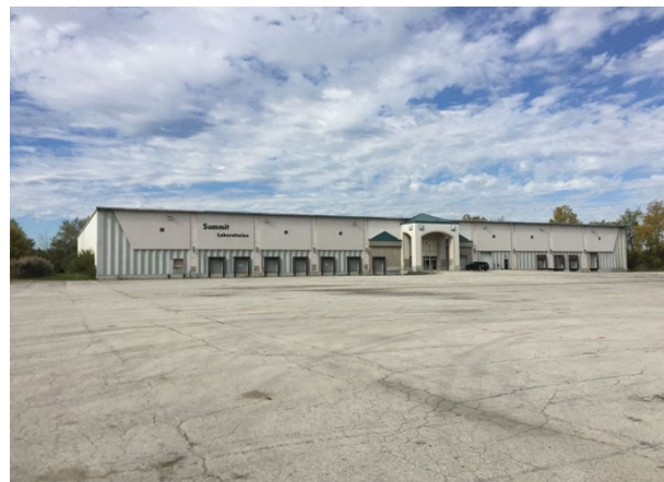
Current photo of the warehouse building.
