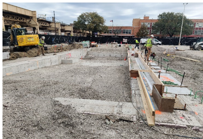
Form work and foundations for the loading dock truck ramp.
