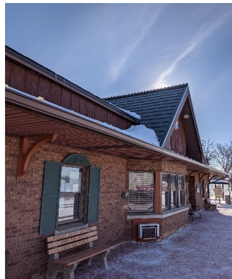
Existing Fox Lake crew facility.
