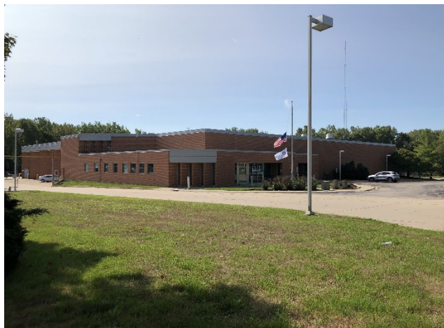
Existing River Division bus garage.
