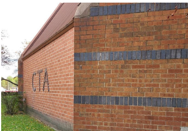
Kedzie Bus Garage façade existing condition.
