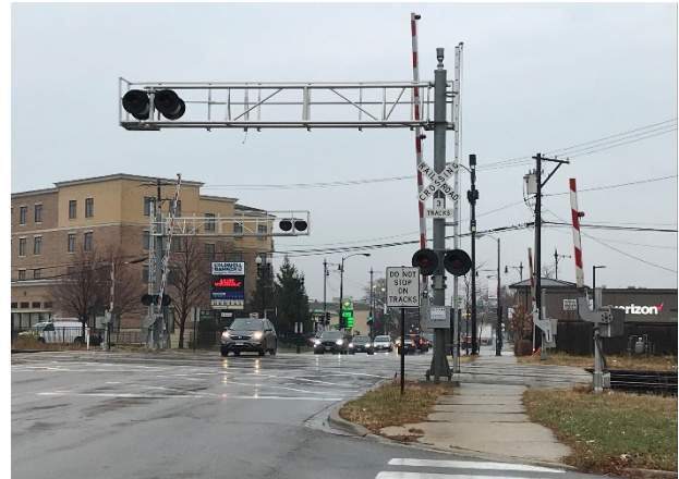
Picture of existing Metra grade crossing.
