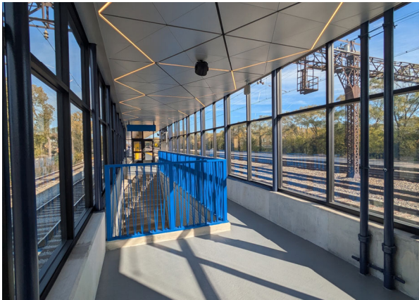
New platform level headhouse at 87 th Street Station.
