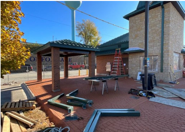
Roofing work at the Fox Lake crew facility.
