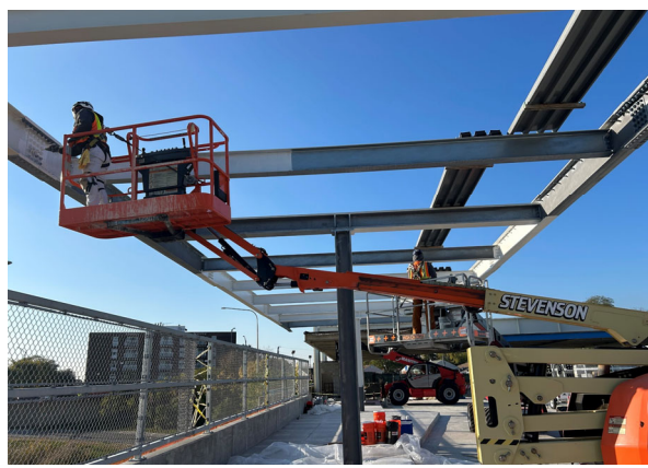
Canopy painting at Harlem Station.
