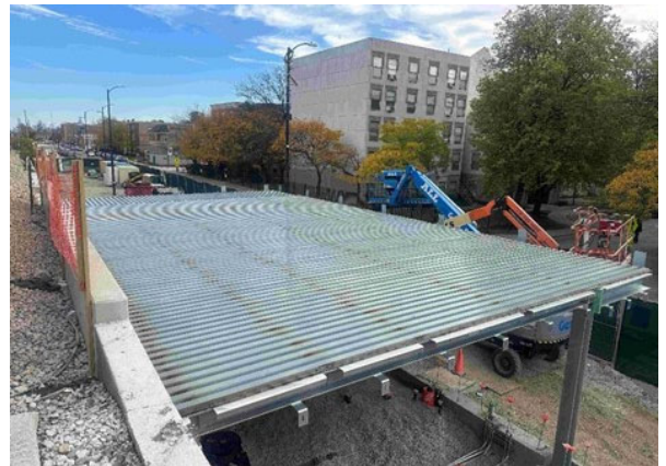
Austin Station roofing steel membrane installation.
