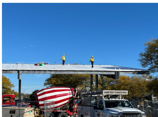
Canopy solar panel installation at North Division Garage.
