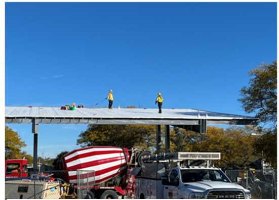
Solar Panel installation at North Division Garage.
