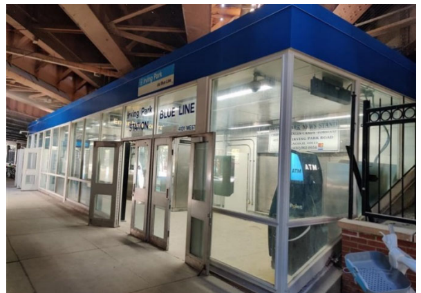
Existing Irving Park Station entrance.
