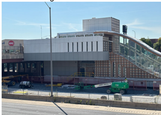
Racine Stationhouse – Bridge Level.
