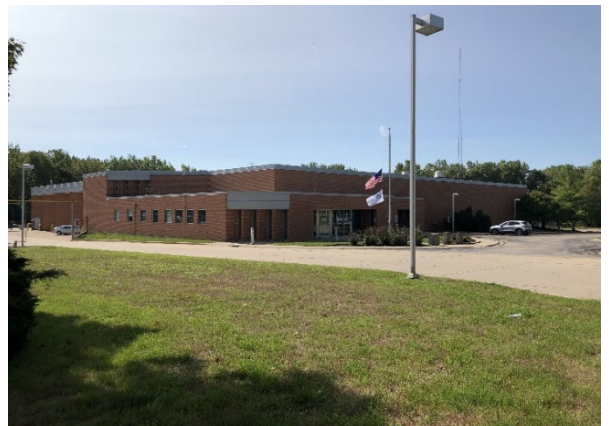
Existing River Division bus garage.
