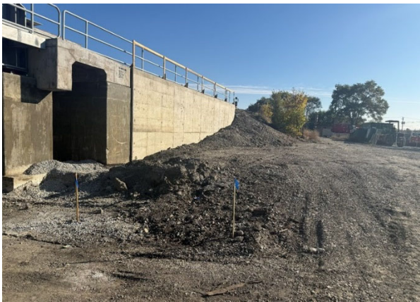
Retaining wall construction at Morgan Street Bridge.
