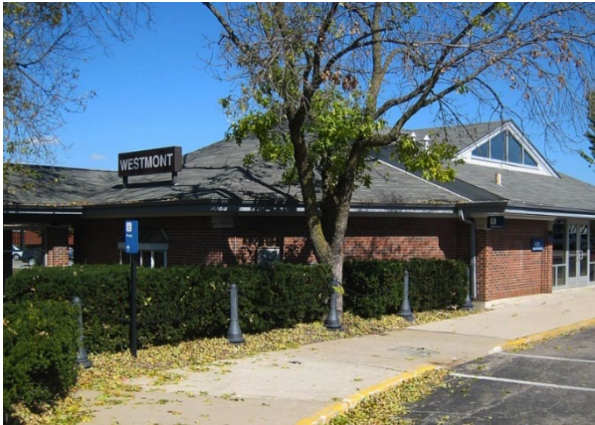
Existing Westmont Station.
