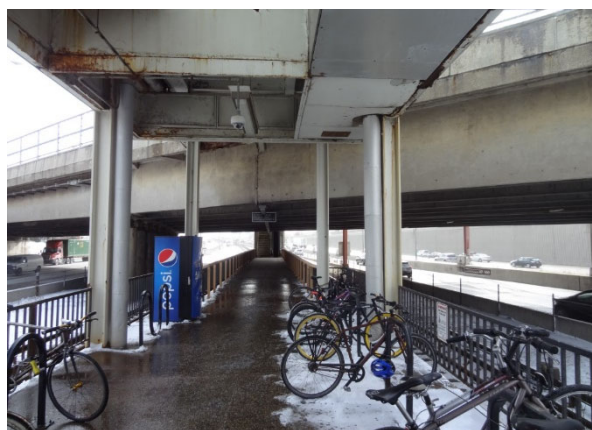
Montrose Station platform – potential placement of elevator.
