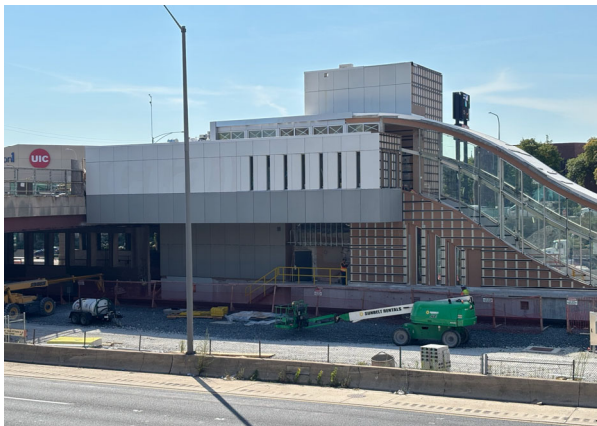
Racine Stationhouse – Bridge Level.
