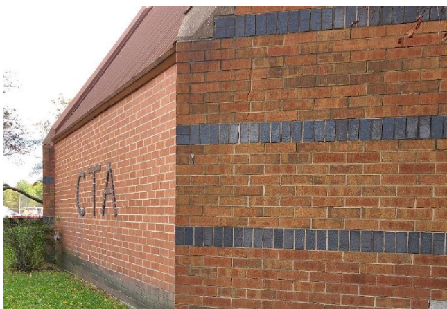
Kedzie Bus Garage façade existing condition.
