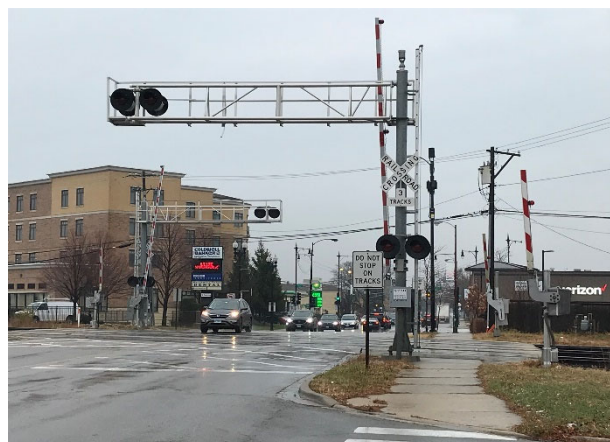
Picture of existing Metra grade crossing.
