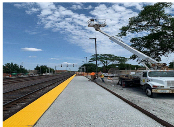
Workers install light fixtures at Melrose Park Station on the UP-West line.
