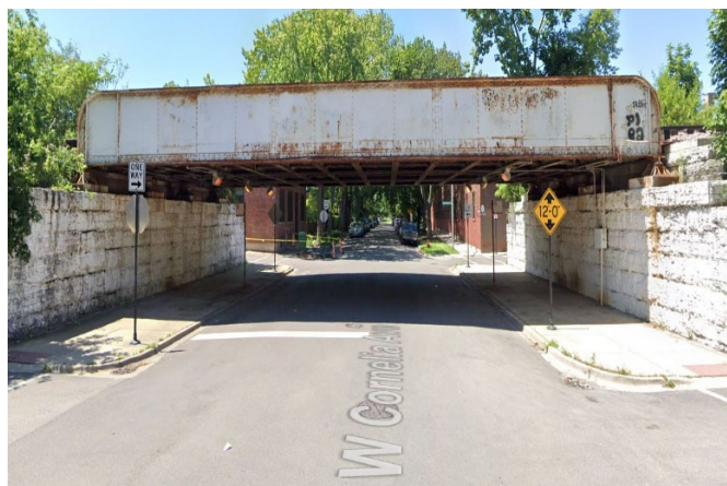
Picture of existing conditions of Cornelia Ave bridge.
